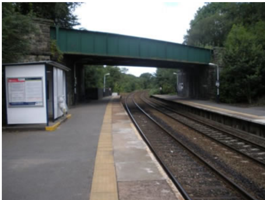
Middlewood Station Bridge
